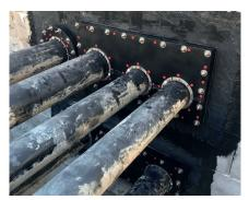
KRASO® Plastic Flange Plate Type KFP multiple with foil flange - Special
