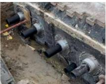
KRASO® Stainless Steel Flange Plate - Special internal diameter: 250 mm, for installation of pipes or cables: 0 to 225 mm using KRASO® Sealing Insert, in front
