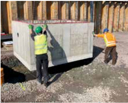
KRASO® Pump Sump - concrete - Special internal dimensions approx. 200 x 270 x 150 cm, external dimensions approx. 250 x 320 x 175 cm, 2 KRASO® Casings Type FE ID 200, made of waterproof concrete, with 25 cm thick, reinforced wall and base plates ( 20 kg per cbm ), rebar connection approx. 8/15 two-rowed, surrounding water pressure tight, MPA-tested construction joint tape KRASOflex® Duo-Fix 150 „plus“, 4 lifting lugs Rd30, weight/piece: approx. 15.30 t, with additional reinforcement according to the indications of the structural engineer
